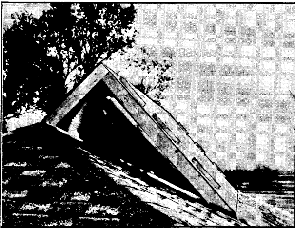
Framing and Sheathing the Collector and Installing Manifolds.
