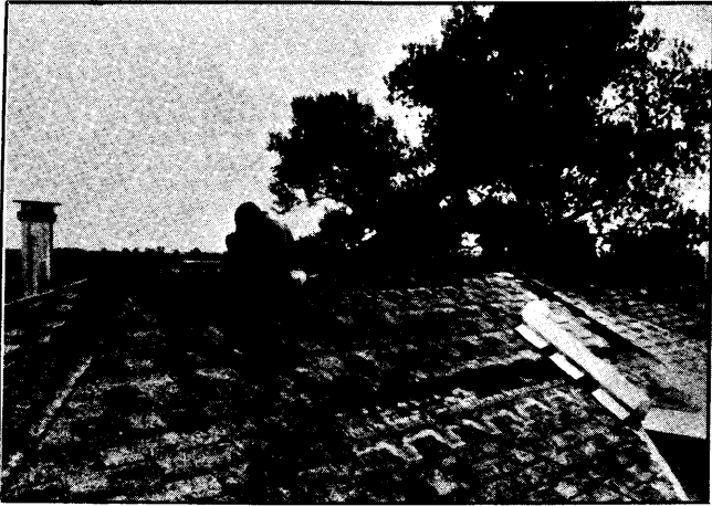
Laying Out the Collector and Removing Shingles.
