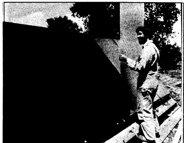
Installing Glazing Supports and Glass.
