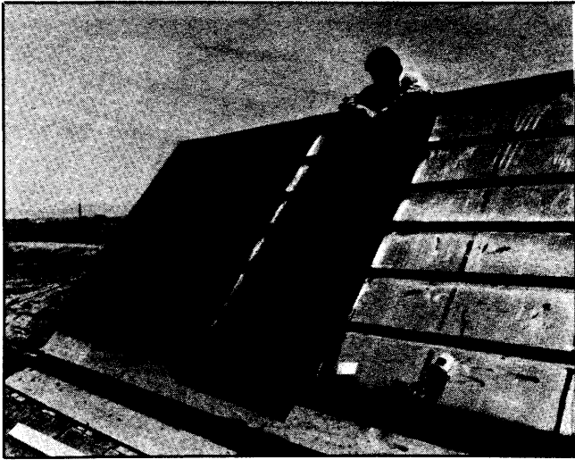
Installing the Insert Absorber Plates.
